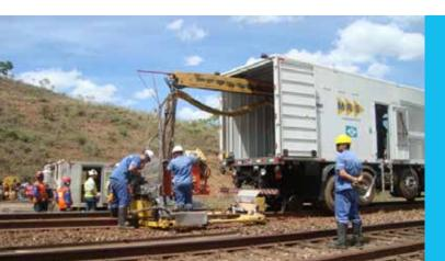
Our MobileWelder® was first introduced to the industry and pioneered by Holland in 1979. This versatile flash-butt welding machine is a virtual mobile welding plant that can travel both on the rail and on the highway and is most easily relocated from one job site to another.
